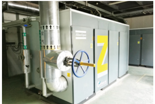
Yixing site WWTP
